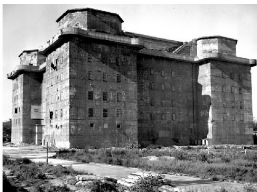
2. The air defense tower (one of three) in Berlin. Each corner (small) tower has a double marine 105 mm. an instrument capable of «getting» an enemy aircraft at an altitude of 14,800 m., or (by firing at ground targets) at a range of up to 22 km., and several 4 \times 4 \times 20 -mm Flak 400 cannons. The towers form a triangle with a side of three kilometers. The roof of the towers is 3.5 m high, reinforced concrete, the wall is 2 m. The building also has a bomb shelter function for the city's population. The Berlin towers are dismantled. Several other buildings (for example, in Hamburg) have been refurbished... either under nightclubs, or shops
